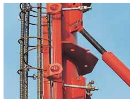
A push-pull prop connection is available on each column panel.
