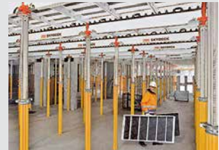
Slab Formwork
