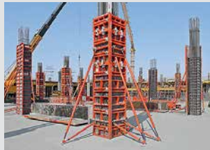
Column Formwork
