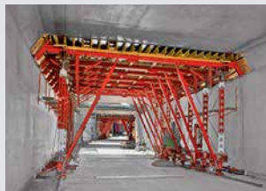
Tunnel Formwork
